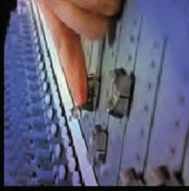
cabina control audiovisual audiovisual control booth
